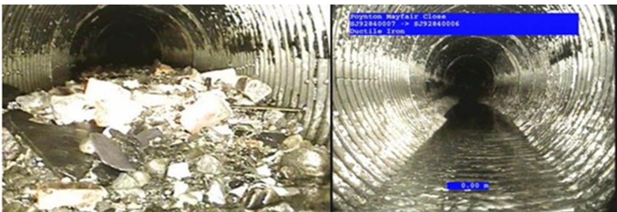
Figure 1 Before and after culverted watercourse cleanse at Mayfair Close
