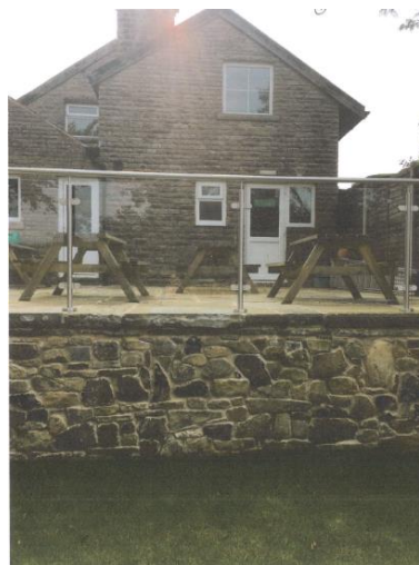
After refurbishment photos
