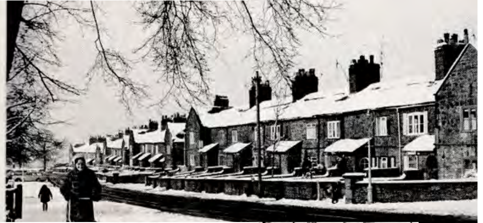
above These stone cottages on Coppice Road were built a hundred years ago for miners. They were constructed, without plans, partly from local stone left over from the building of the steeple for St. George's Church.
