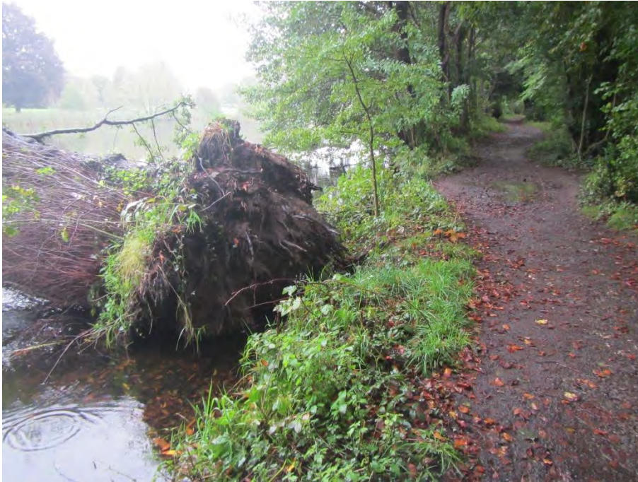
Photo 5 – Fallen Tree along Upstream Face
