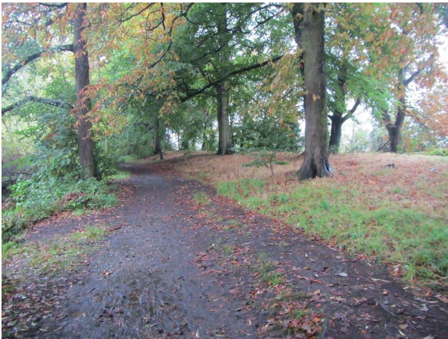
Photo 6 – Broad Crest Dam south of the Overflow
