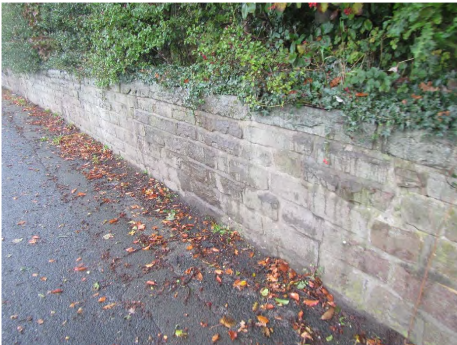
Photo 10 – Central Section of Masonry Wall
