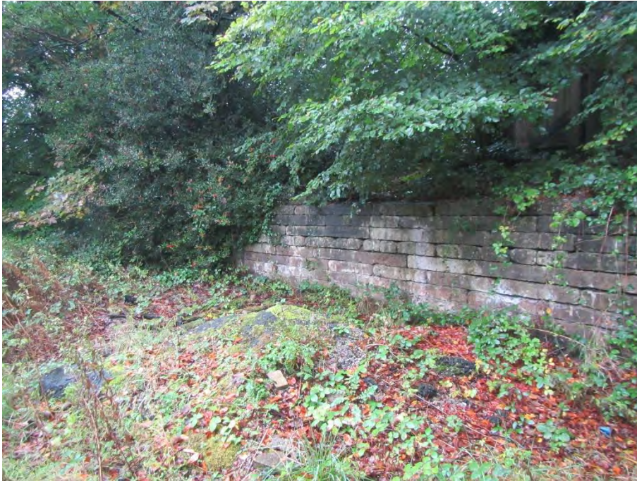
Photo 9 – Masonry Retaining Wall within the Old Council Depot
