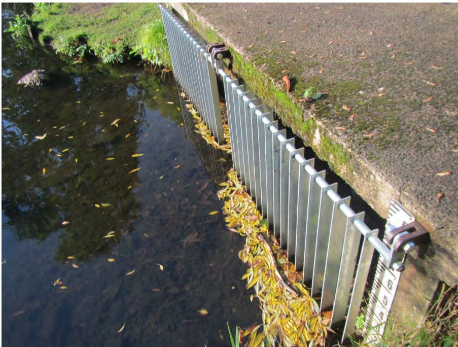
Photo 2 – Inlet structure with new screen at the upstream end of the overflow pipe
