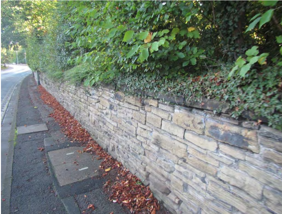
Photo 8 – Masonry Retaining Wall within the Old Council Depot
