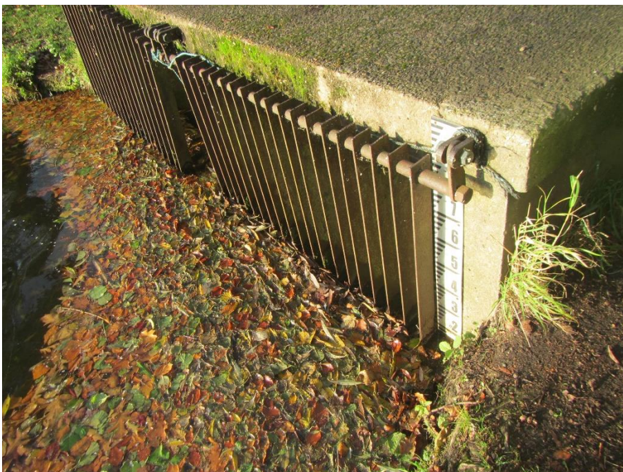
Photo 2 – Inlet Structure with Screen at the Upstream end of the Overflow Pipe
