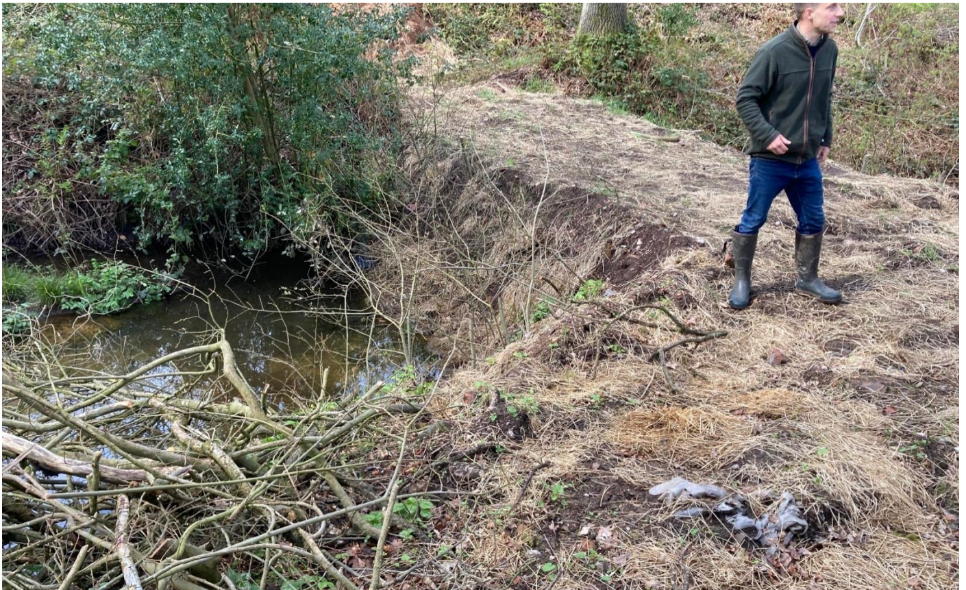
Clay bund at the Gables
