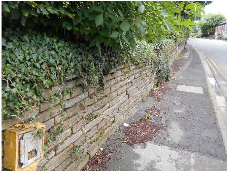
Photograph A7: Masonry retaining wall alongside the A523
