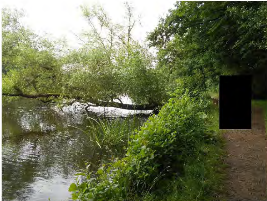
Photograph A3: Fallen tree at the upstream face
