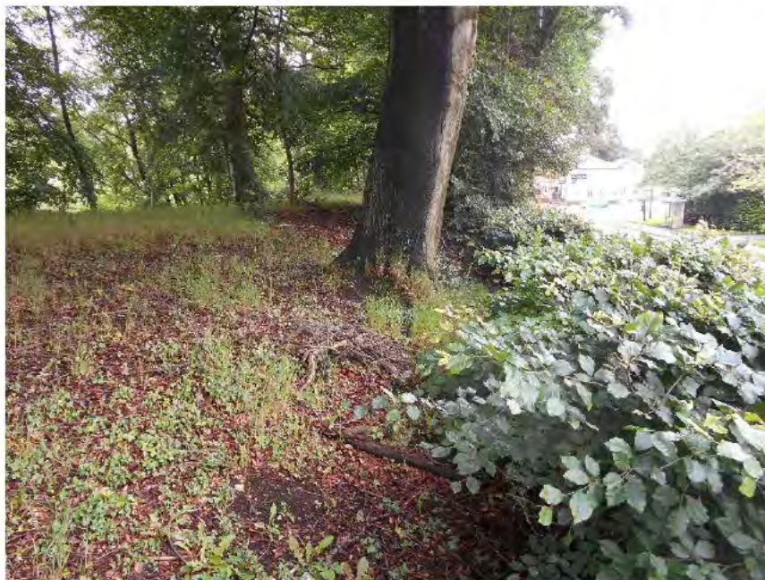
Photograph A6: Typical slope of the downstream face above the wall
