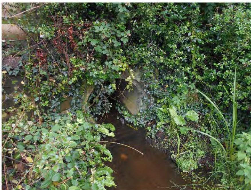
Photograph A13: Inlet pipe to reservoir at southern end (Poynton Brook)
