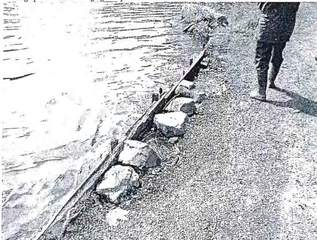
Photograph 2 – Timber edging and stone on upstream face
