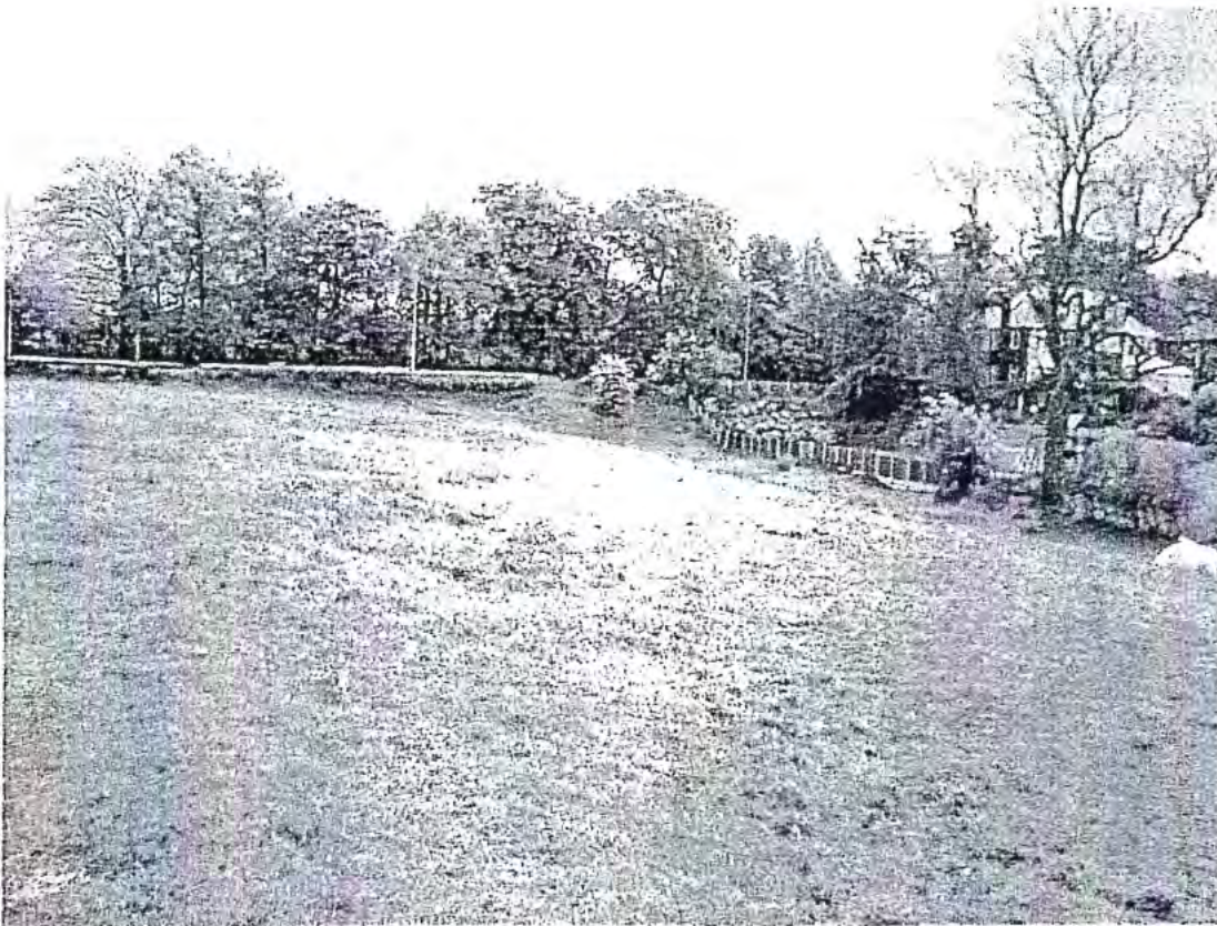
Photograph 11 – Downstream slope at highest point
